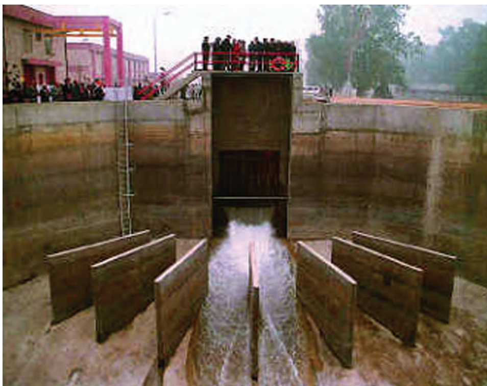
Fig. 18.10 : Water treatment plant
